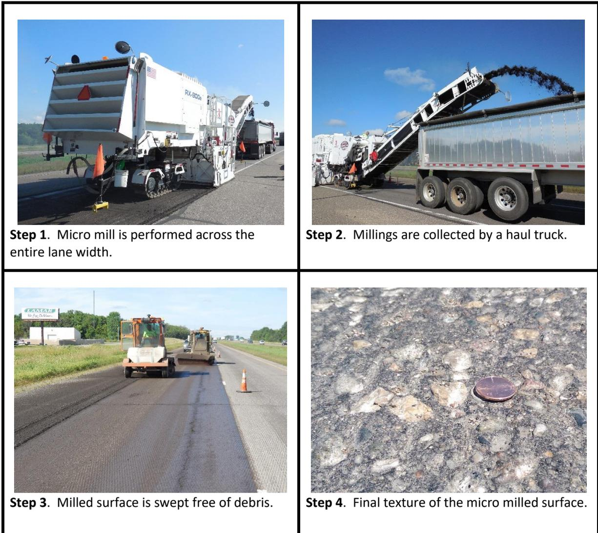
**Figure 4.12: General Micro Mill Construction Steps**
