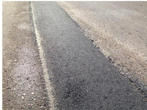
Patched area after compaction with steel drum roller.
