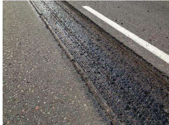
Milled area with tack coat prior to patching.
