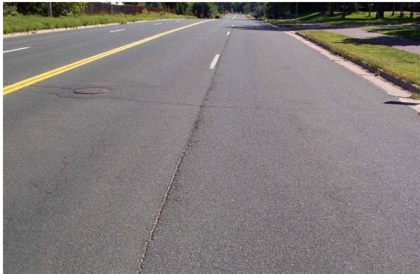
**Figure 5.00 Low Severity Longitudinal Joint Deterioration**
