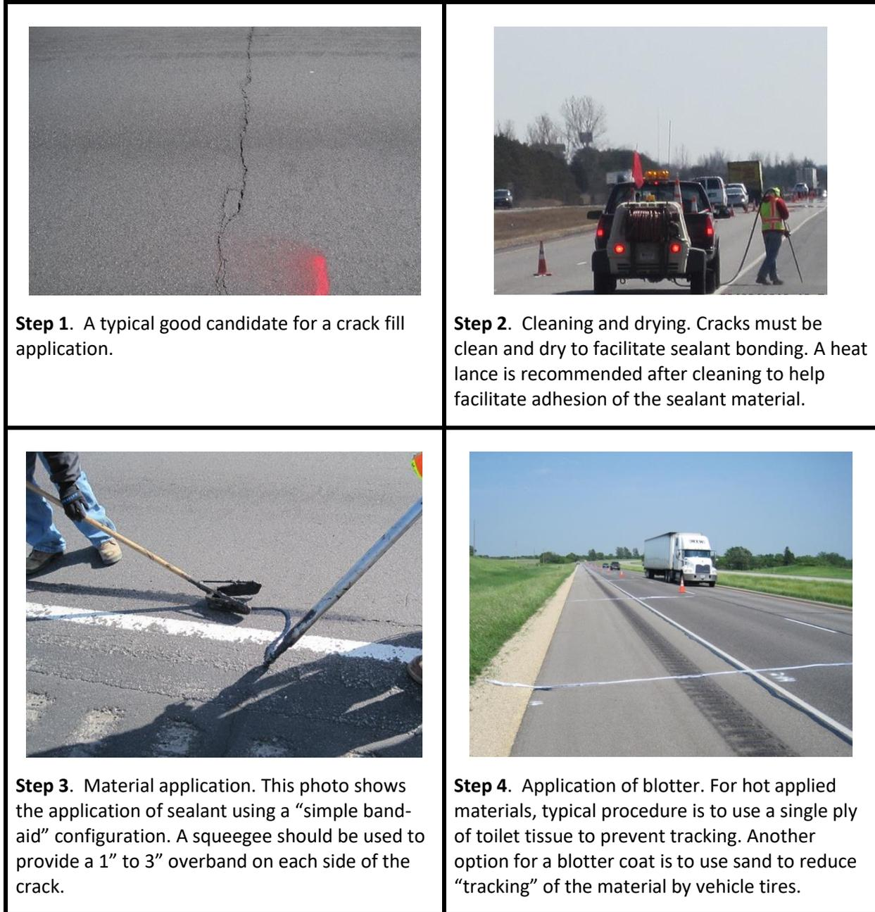
**Figure 4.03: General Crack Fill Construction Steps**
