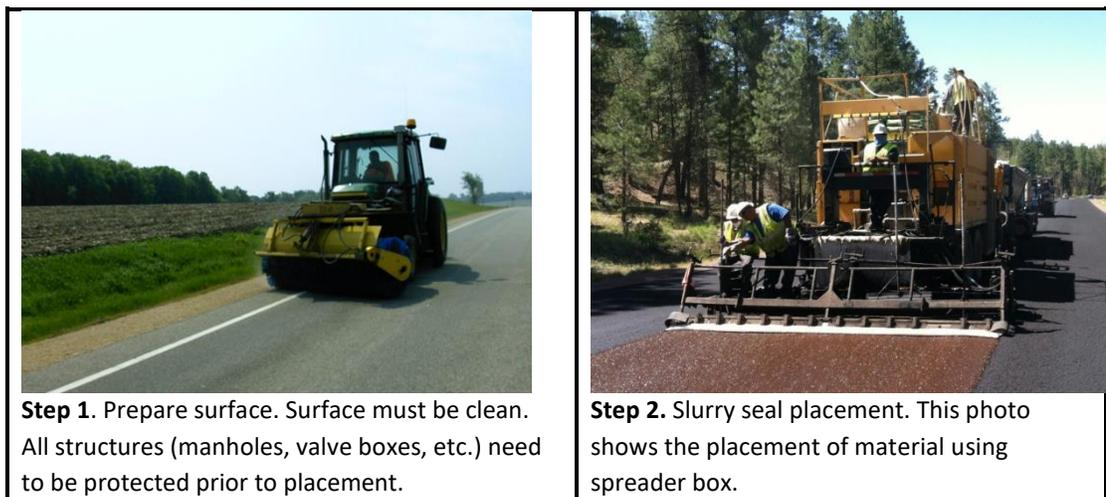
**Figure 6.05: General Slurry Seal Construction Steps**
