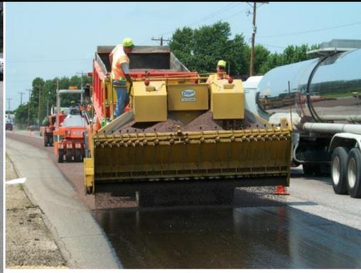
**Step 3.** Chips are spread from a self-propelled, pneumatic tired unit onto the roadway.
