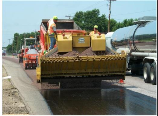
**Steps 2 & 3.** Emulsion and chip application. The asphalt emulsion is applied to the surface with a distributor truck. Chips are spread from a self-propelled, pneumatic tired unit with a hopper on the front from which the chips are placed onto the roadway
