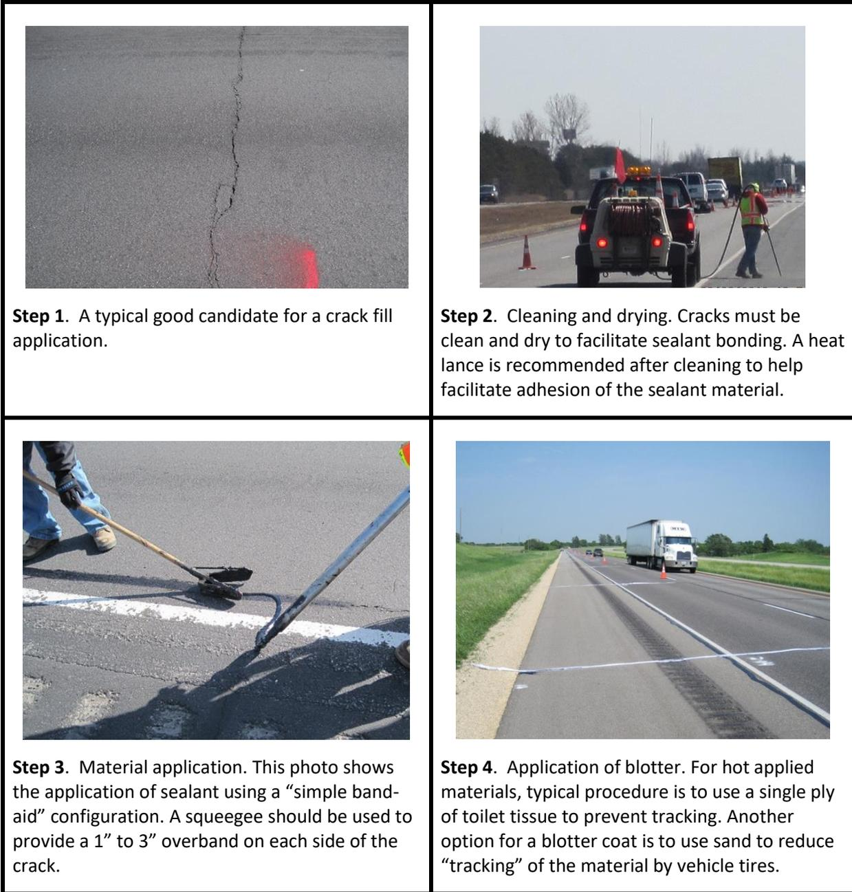
**Figure 4.03: General Crack Fill Construction Steps**
