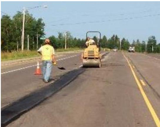
Asphalt is placed into the milled area and compacted with a steel drum roller.
