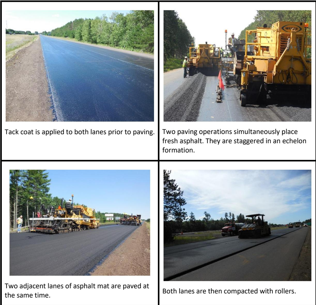
**Figure 5.08 Echelon Paving**
