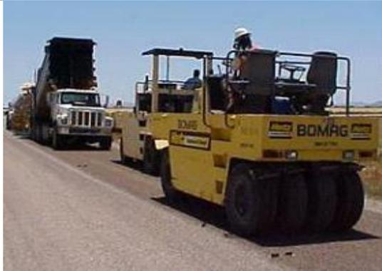
**Steps 4 & 5.** Rolling and sweeping. After the application of the aggregate, the surface is rolled with pneumatic tired rollers and swept to remove excess aggregate.
