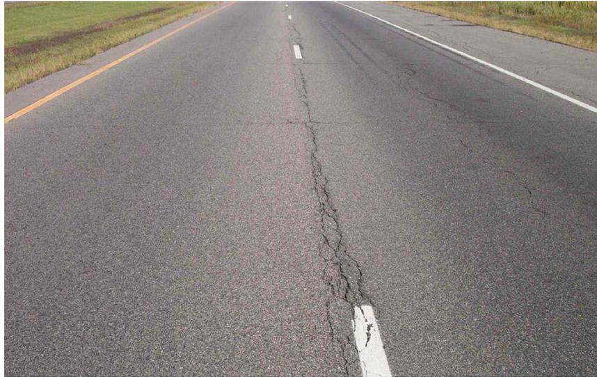
**Figure 5.01 Medium Severity Longitudinal Joint Cracking**
