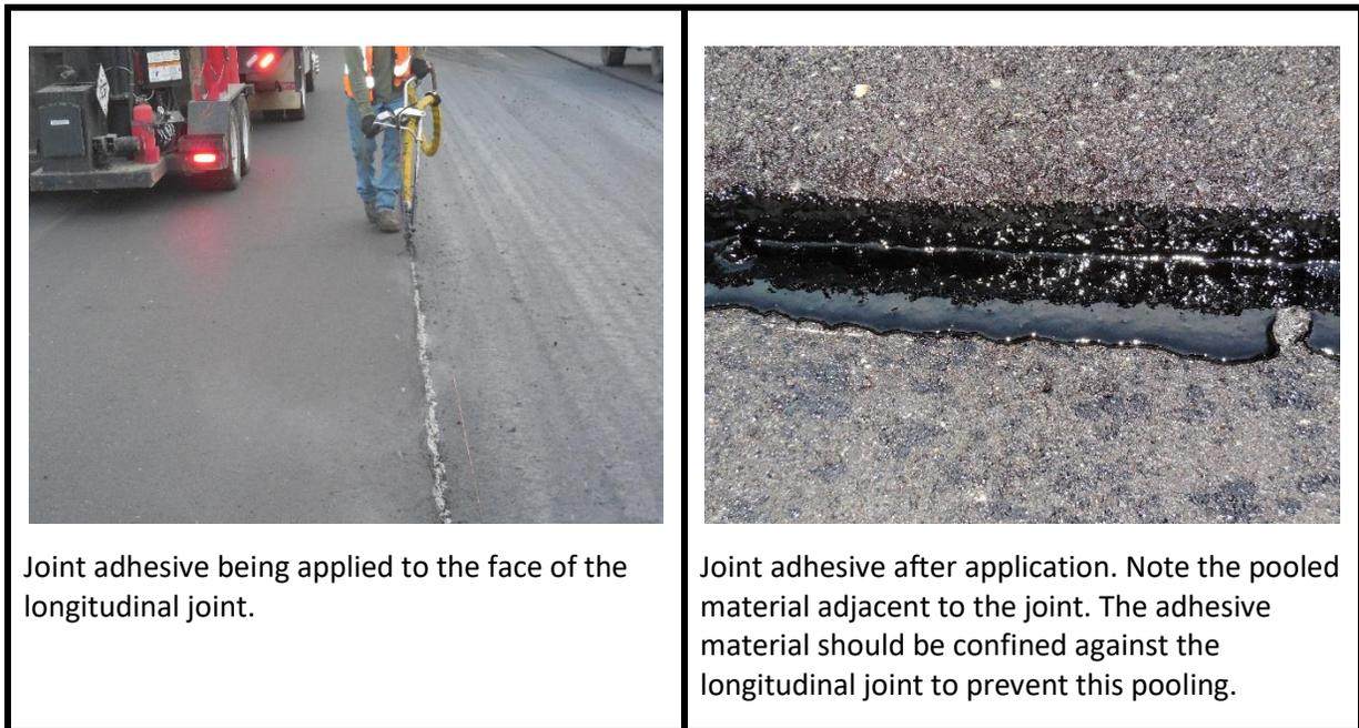
**Figure 5.10 Joint Adhesive Application**
