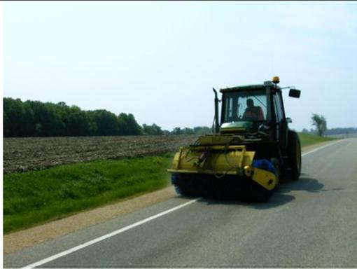
**Step 1.** Prepare/clean surface. All structures (manholes, valve boxes, etc.) need to be protected prior to placement. Striping may be pre-treated with emulsion.
