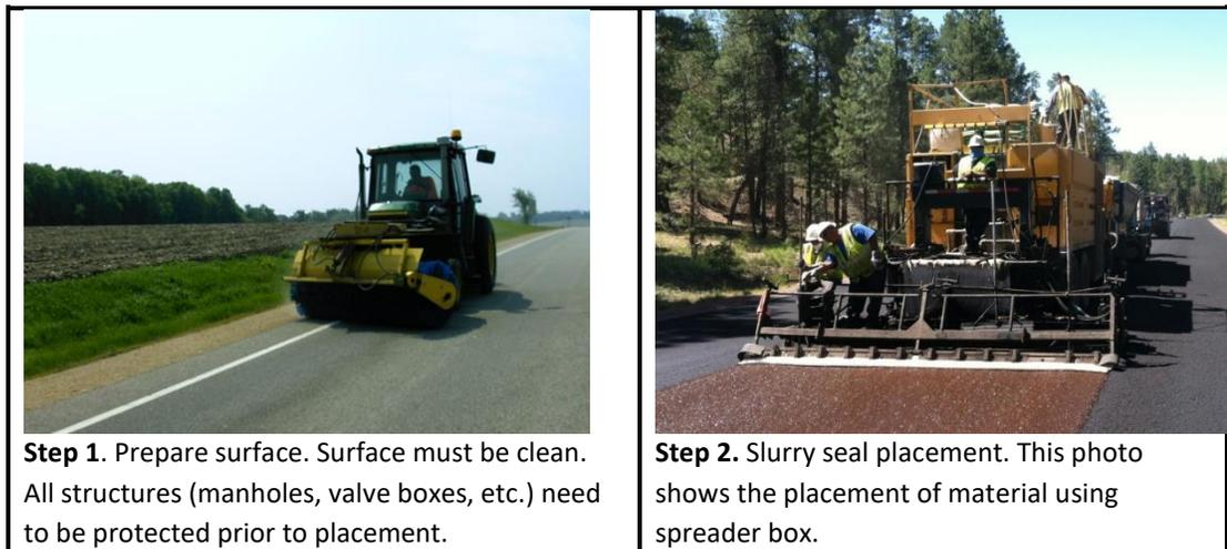
**Figure 6.05: General Slurry Seal Construction Steps**
