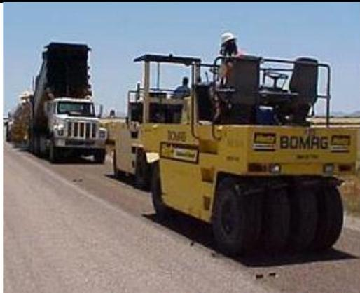
**Step 4-5.** Rolling and sweeping. After the application of the aggregate, the surface is rolled with pneumatic tired rollers and swept to remove excess aggregate.
