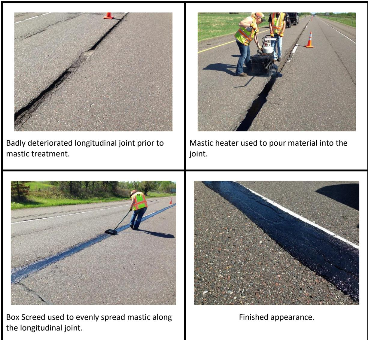
**Figure 5.03 Longitudinal Joint Treatment with Mastic**
