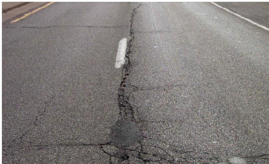
**Figure 5.02 High Severity Longitudinal Joint Cracking**
