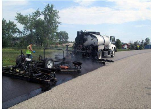
**Step 2** The asphalt emulsion is applied to the surface with a distributor that pulls a sled that houses a series of brooms placed at different angles. These brooms guide or "scrub" the emulsion into cracks.
