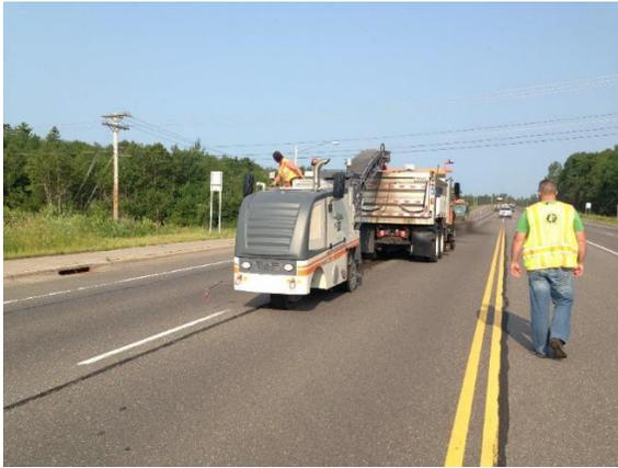
A small mill is used to prepare the longitudinal joint for patching.
