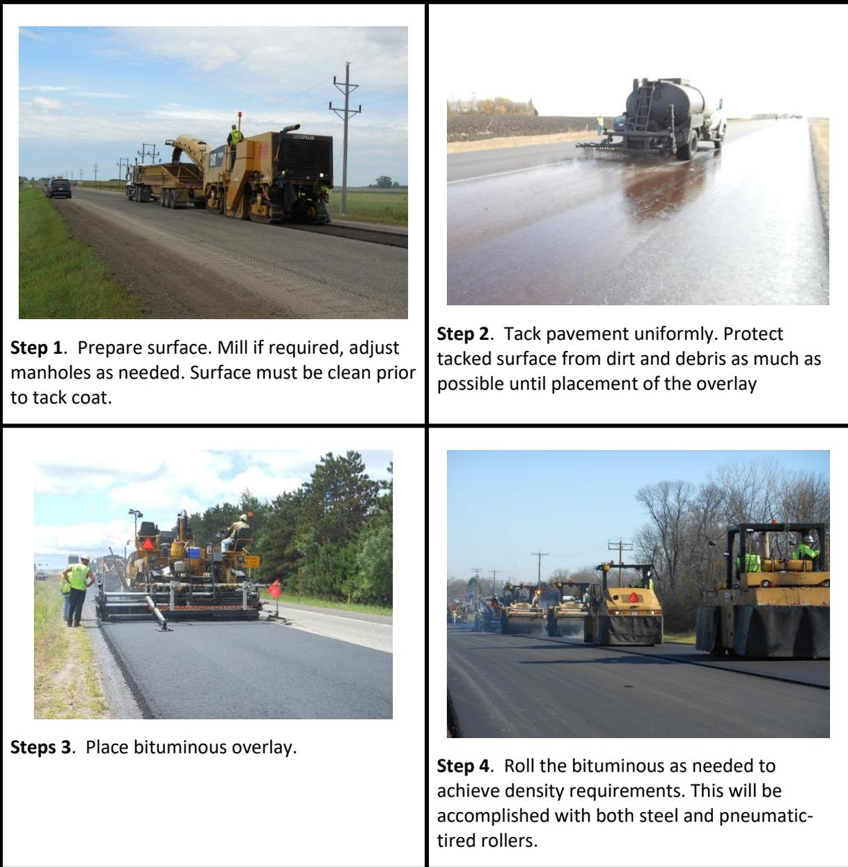
**Figure 4.11: General Thin Lift Overlay Construction Steps**
