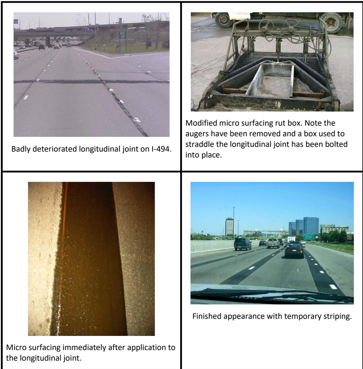
**Figure 5.04 Micro Surfacing of Longitudinal Joints**
