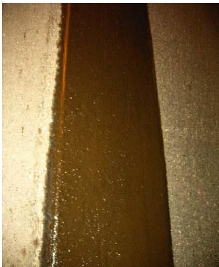
Micro surfacing immediately after application to the longitudinal joint.
