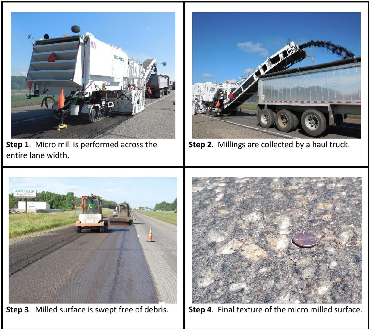
**Figure 4.12: General Micro Mill Construction Steps**
