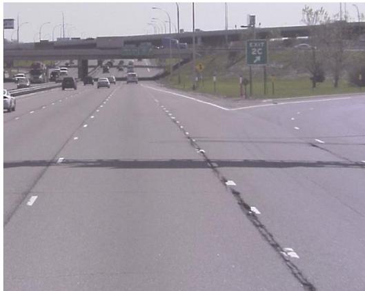
Badly deteriorated longitudinal joint on I-494.
