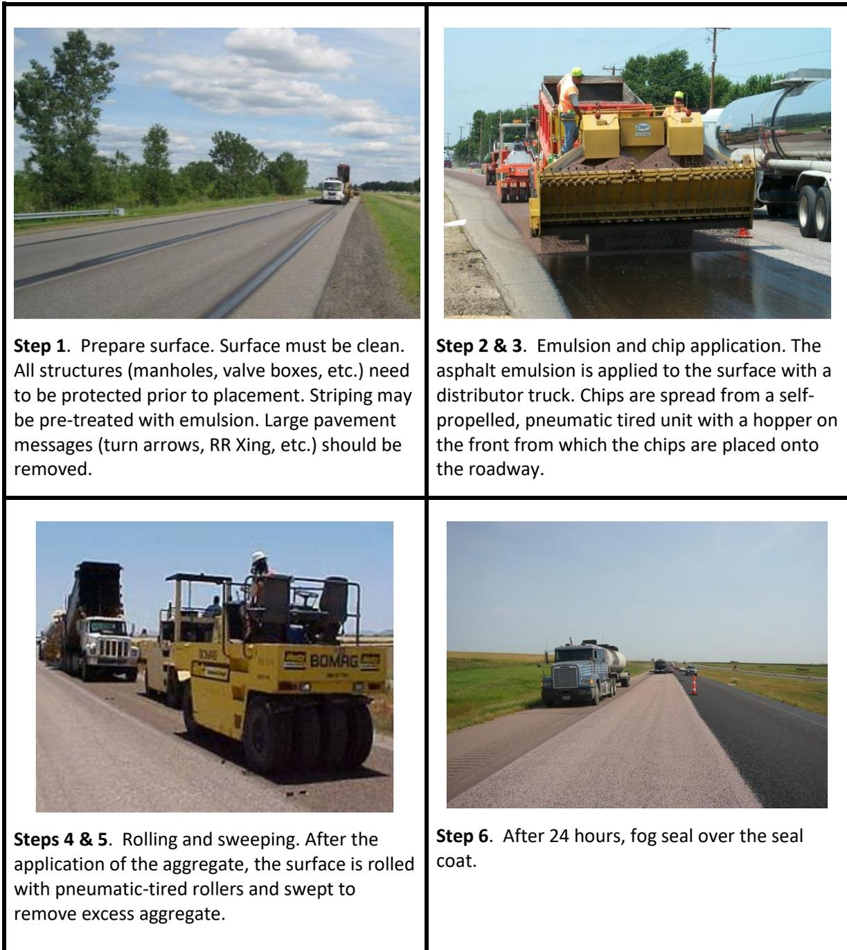
**Figure 4.07: General Seal Coat Construction Steps**
