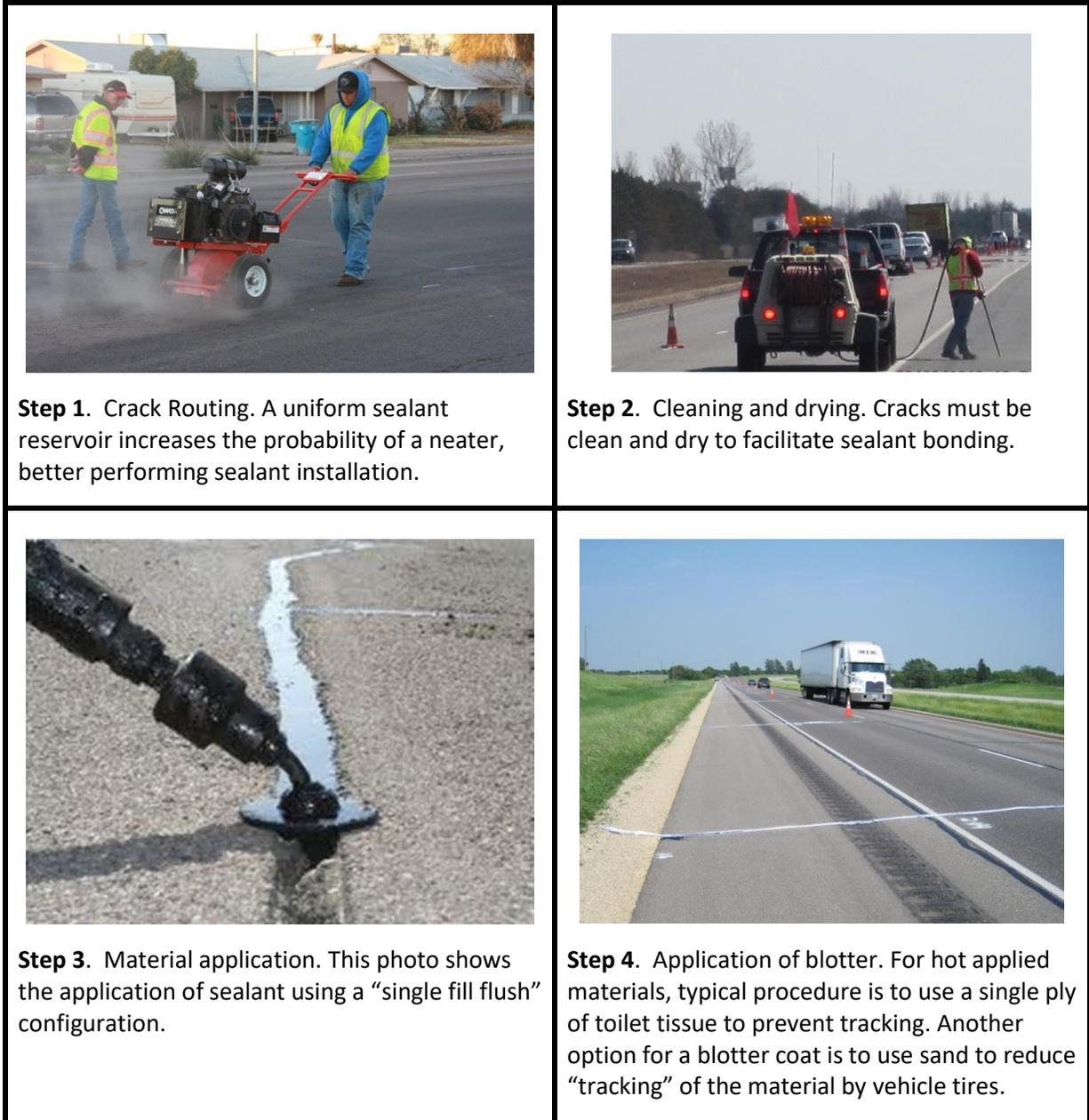
**Figure 4.04: General Rout and Seal Construction Steps**
