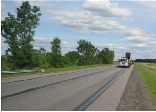
**Step 1.** Prepare surface. Surface must be clean. All structures (manholes, valve boxes, etc.) need to be protected prior to placement. Striping may be pre-treated (as shown here) with emulsion. Large pavement messages (turn arrows, RR Xing, etc.) should be removed.
