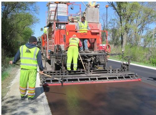
**Step 7.** Micro surfacing placement. This photo shows the placement of material using a micro surfacing spreader box.
