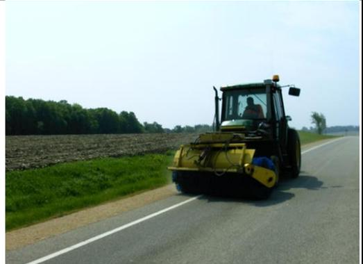
**Step 6.** Prepare surface. Surface must be clean. All structures (manholes, valve boxes, etc.) need to be protected prior to placement.
