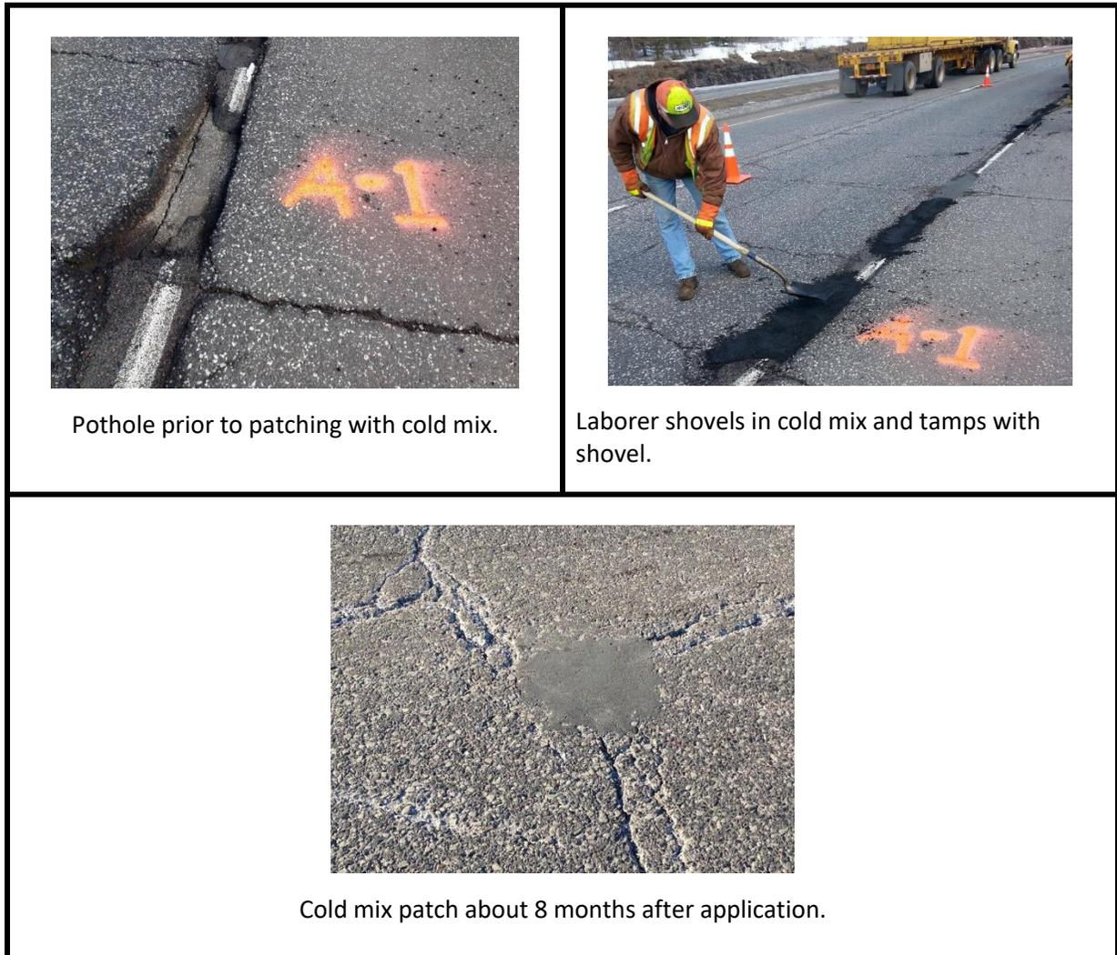
**Figure 5.05 Cold Mix Hand Patching**
